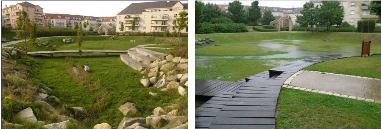
Creation of a floodable garden to manage rainwater in the Clos Saint Vincent district, Noisy-le-Grand. © Département de Seine-Saint-Denis
