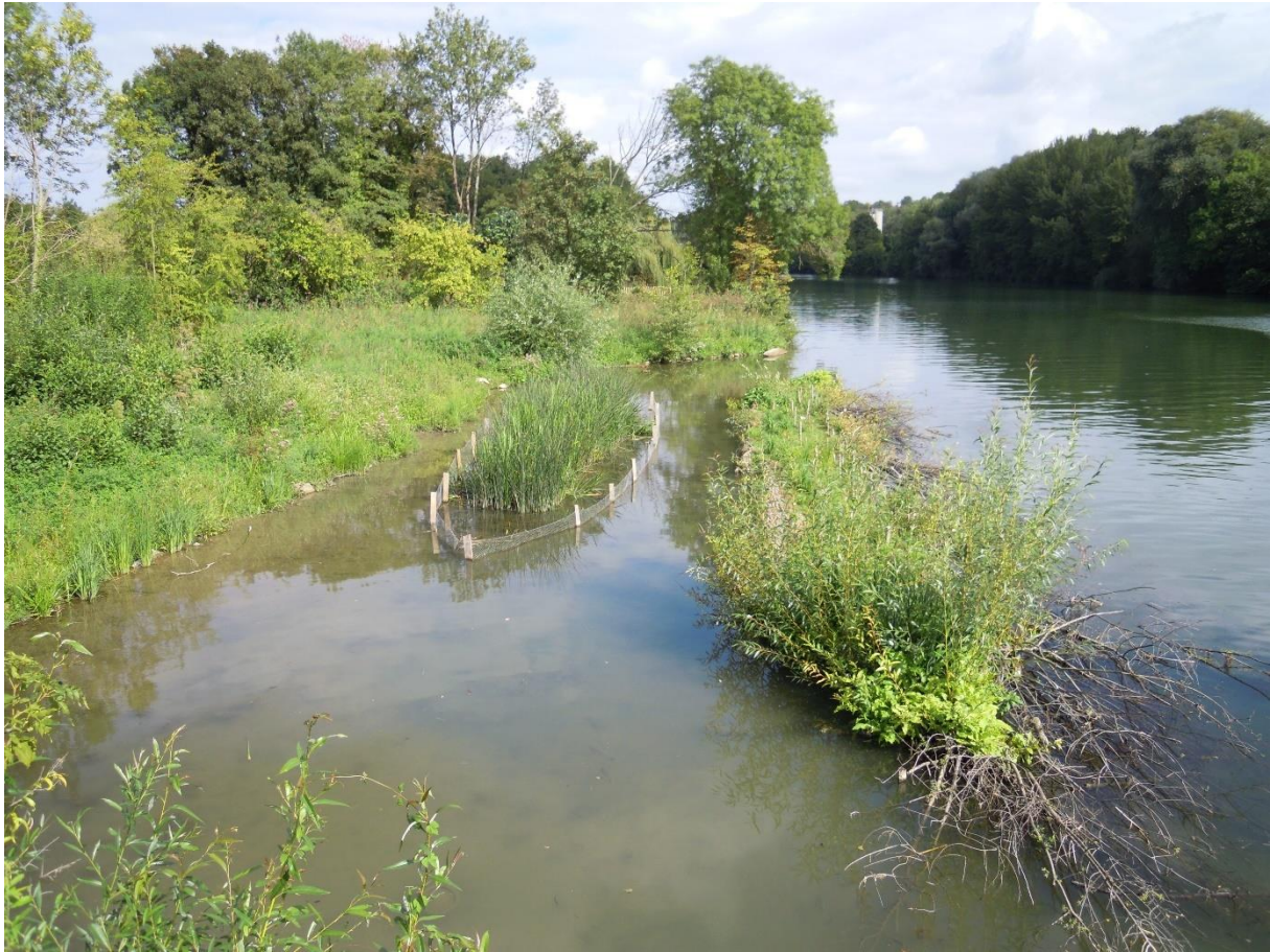
Ecological engineering techniques used to restore the banks in order to protect them from erosion, stabilise them and allow them to regenerate. ©Gilles Lecuir
