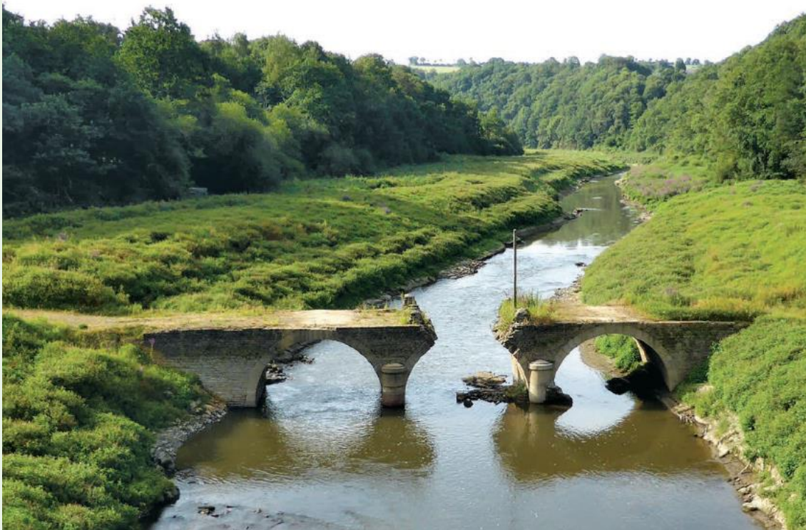
Spontaneous renaturing of the banks of the Sélune, 2 years after gradually emptying two dams and reshaping the banks. ©Charlotte Ravot
